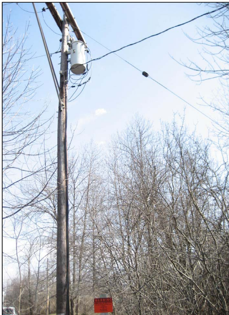
Photograph 1: Pole-type transformer along wooded area.
